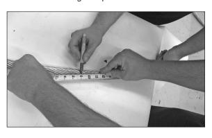
Step #5 Measure from the "Press First" Knurl in the middle of the galvanized steel splice tube to the end. Add 1" to this length to allow for aluminum strand expansion when the splice tube is applied. Mark this length ("cutting length") on the conductor to cut back
