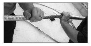
**Step #19** Center the aluminum splice body over the two pieces of conductor and the steel core splice tube.
