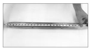
**Step #4** Measure and mark half this length on the conductor from the cut strand ends. This will be important later when centering the splice.
