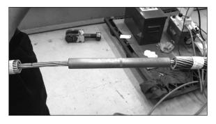
NOTE: THE STEEL CORE OF THE CONDUCTOR MUST BE FULLY INSERTED INTO THE STEEL CORE SPLICE TUBE. FAILURE TO PROPERLY FILL AND COMPRESS THE CORRECT LENGTH OF THE STEEL CONDUCTOR CORE WITHIN THE STEEL CORE SPLICE TUBE IS A MISAPPLICATION OF THE PRODUCT.
