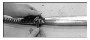
**PLP TIP:** If any difficulty is encountered sliding the aluminum splice body over the second piece of conductor, the aluminum strand ends can be filed again to remove burr. Also, to compress or make the strands more concentric, a small hose clamp may be applied temporarily while the tube is slid over the aluminum strand ends.
