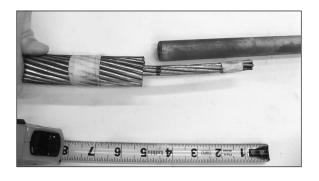
Step #9 Apply the aluminum splice body over the conductor, pushing it completely through the other end before compressing the steel core splice.
