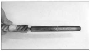
Step #12 Setup the other piece of conductor to be spliced by repeating the conductor preparations found in Steps 3 through 8, 10 & 11. Once complete, fully insert the second conductor's steel core into the steel splice tube. Make sure that both cores are now fully inserted to the middle of the splice tube near the "Press First" knurl with the ends of the steel tube falling at the marks made on the conductor core.
