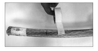
**Step #7** Cut the outer aluminum strands at the cutting mark to expose the steel core.
