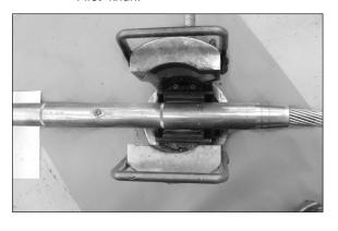
Step #26 Starting at the "Press First" knurl, compress the aluminum splice body over the conductor, applying compressions first at the knurl and working all the way to the end of the aluminum tube.
