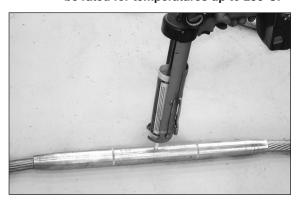
**Step #21** Cease application when filler compound seeps out the tapered "conductor facing" end of the hardware.
