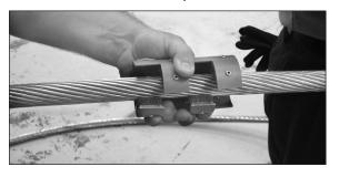
Step #2 Remove the plastic plug from the aluminum body. Inspect the inside bores of the hardware to ensure that there are no sharp points or other defects.
