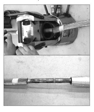
Step #18 Slide the aluminum splice body towards the steel core splice tube. When the edge of the tube is close to the taped strand areas, remove the tape as the aluminum splice tube will now hold the conductor strands in place.
