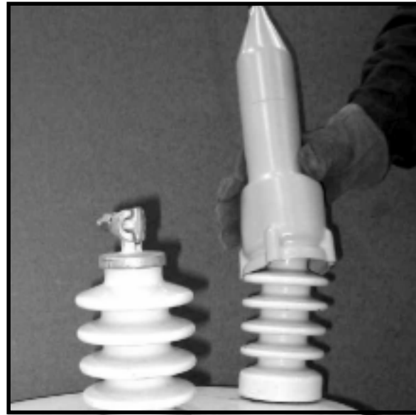
FIGURE 6 - Installing WP on the bushing
