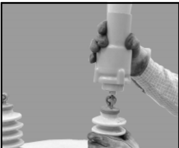
FIGURE 9 - Installation of base
