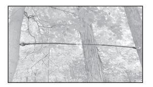
**PLP Tip:** Install the TREE-GRIP<sup>™</sup> Dead-end, thimble, and cable. Reference the TREE-GRIP Dead-end application procedure (SP2056).
