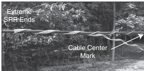
FIGURE 6: LEFT SRR SET OF A TWO-SET APPLICATION. FIRST ROD APPLIED FROM THE CABLE CENTER MARK OUTWARD SUBSEQUENT RODS ALIGNED AT EXTREME END AND WRAPPED INWARD TOWARD CENTER.
