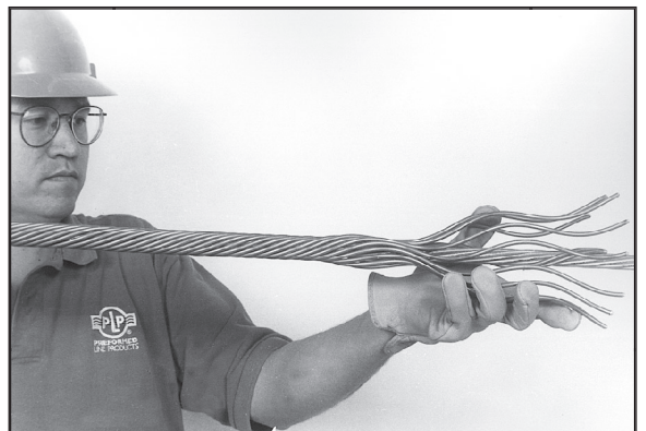
FIGURE 20: WRAP ROD ENDS IN PLACE
