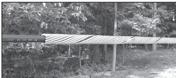
FIGURE 7: LEFT SRR SET COMPLETED AND ROD ENDS ALIGNED.
