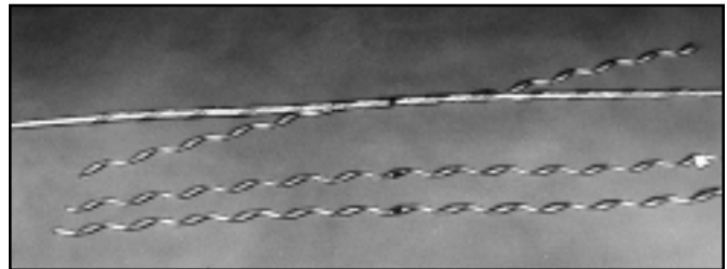
FIGURE 4 - APPLY ONE TO TWO PITCH LENGTHS OF SECOND SUBSET
