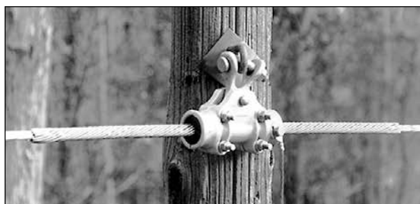
FIBERLIGN Cushion Clamp installed
