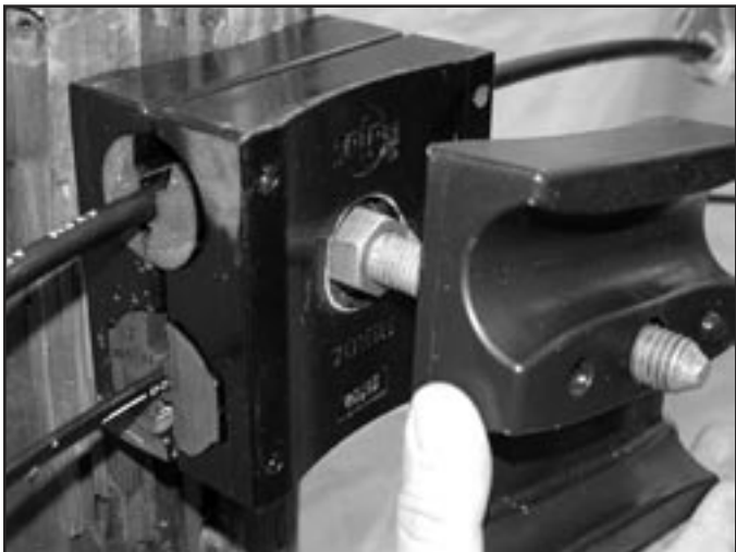
FIGURE 12 - SECOND FLS INSTALLATION AGAINST THE FIRST
