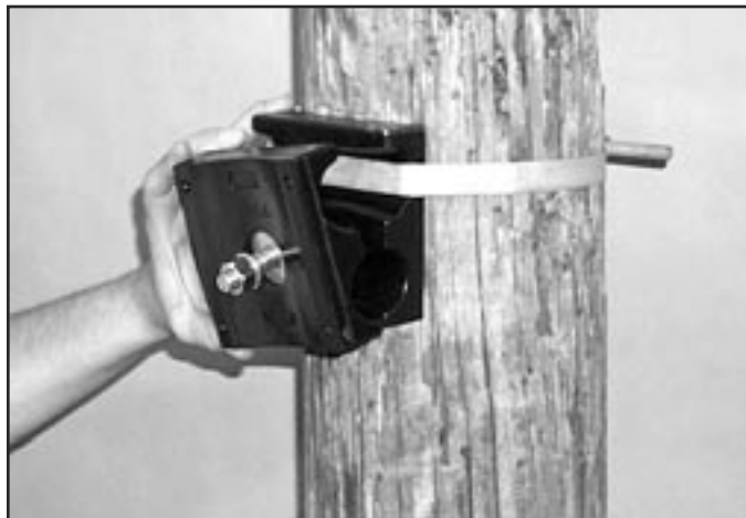
FIGURE 9 - INSTALL NUT AND LEAVE HOUSINGS LOOSE
