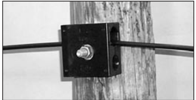
FIGURE 13a - STRINGING THROUGH LARGE CAVITY
