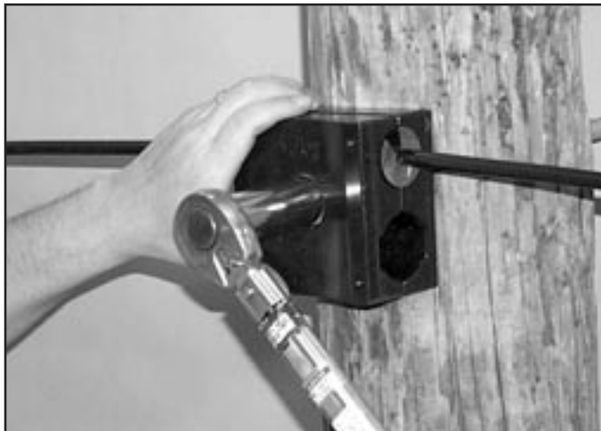
FIGURE 6 - TORQUE TO 30 FT-LB
