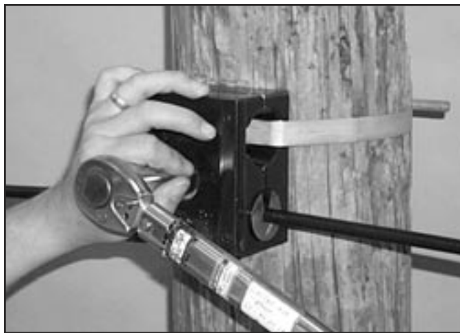
FIGURE 10 - TORQUE TO 30 FT-LBS (41Nm)
