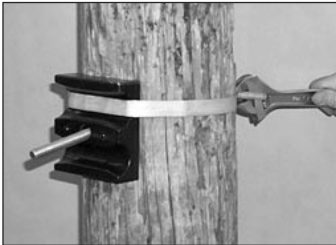
FIGURE 8 - BAND HOUSING HALF TO POLE
