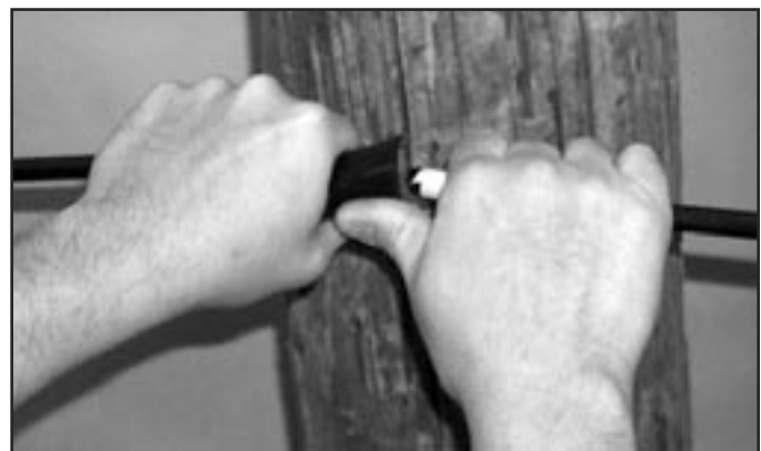
FIGURE 4 - ONE HAND SQUEEZES CABLE INTO INSERT AND THE OTHER HAND SUPPORTS THE CABLE AND PRESSES INSERT WITH THUMB
