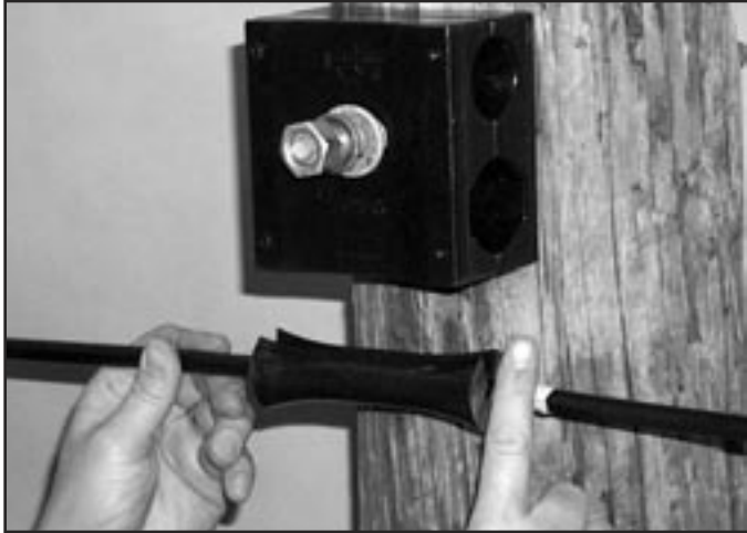
FIGURE 5 - ORIENT AND INSERT WITH SLOT UPWARD
