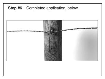
**NOTE:** C-Rural Dead-ends are specifically designed for use with high density polyethylene coated wire.
