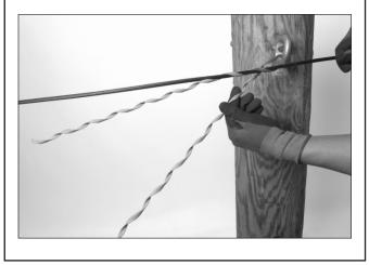
**Step #4** Apply both legs by pulling out and away from wire.
