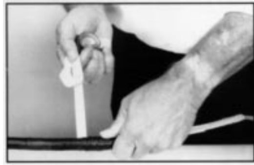
FIGURE 13 – APPLYING LOCK-TAPE SEALANT
