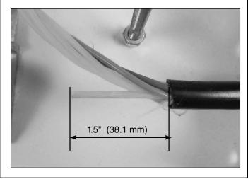
Step #13 Position the strength member of the cable under the cap of the strength member bracket and tighten the nut to secure the strength member.
