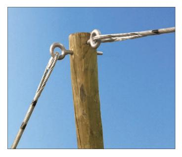
**Wire Rope Dead-ends** are designed for use in agricultural construction of galvanized steel wire rope and EHS strand. Ideal for guying to ground anchors or spanning pole-to-pole, the dead-end loop is manufactured to fit all appropriate hardware.
