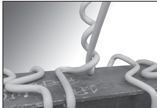
**Step #6** Continue wrapping the helical leg until it is completely installed.
