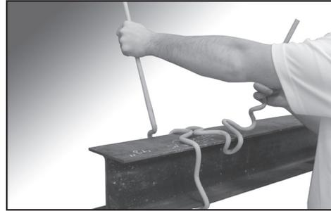
**Step #4** Install a second BIRD PERCH DETERRENT in the same manner as in Steps 1-3. Install the second BIRD PERCH DETERRENT with the uprights oriented the same way as the first BIRD PERCH DETERRENT.
