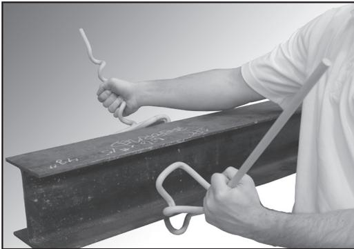
**Step #2** Keeping the uprights of the BIRD PERCH DETERRENT apart, position the unit so that the hooks are over the top of the I-Beam.
