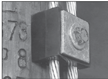
FIBERLIGN Downlead Cushion mounted to wood pole
