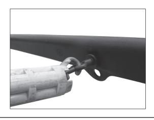
Step #7 Completed installation of the RPC for vertical trunnion mount insulator.
