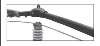
Step #5 Snap both legs of the RPC over the conductor.
