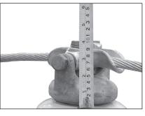
Step #3 Cut the RPC on the appropriate cut line. Ensure that the cut is straight along both lines on either side of the RPC.
