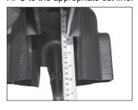
**Step #4** Next place the RPC over the center of insulator and conductor.
