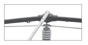
Step #5 Apply pressure to the top of the RPC using the hot stick and completely snap it over the conductor. Another stick can be used to snap the legs into place.
