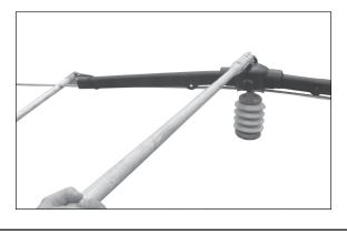
Step #6 Install the four Round Eye Lock Pins included, using the hot stick.
