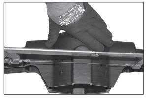
Step #2 Using that measurement, measure from the inside center location of the RPC to the appropriate cut line.
