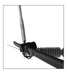
Step #5 Apply pressure to the top of the RPC using the hot stick and completely snap it over the conductor. Another stick can be used to snap the legs into place.
