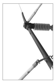
Step #6 Install the four Round Eye Lock Pins included, using the hot stick.
