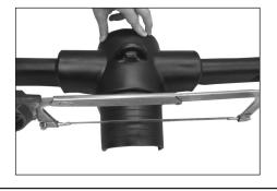
**Step #4** Next place the RPC over the center of insulator and conductor.
