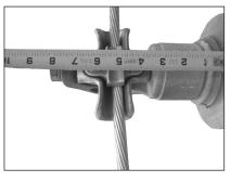
Step #2 Using that measurement, measure from the inside top location of the RPC to the appropriate cut line.
