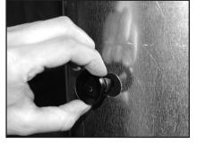
Step #2 Insert the POLE PLUG into the hole, and push until the POLE PLUG is completely installed in the hole.
