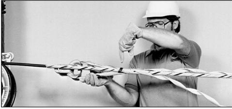
**STEP 8** Continue the installation by wrapping the leg(s) around the SRL as shown below. Whether you wrap one leg at a time or both simultaneously, make sure the gap between both legs is evenly spaced.
