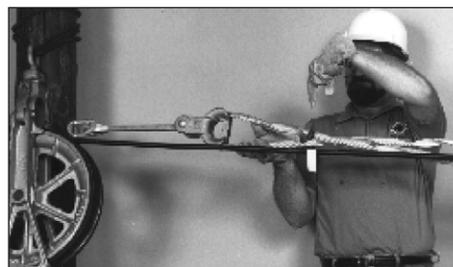
**STEP 2** Mark the cable at the color-coded crossover mark on the dead-end. This will be the reference mark for positioning the structural reinforcing layer (SRL) subsets on the cable.
