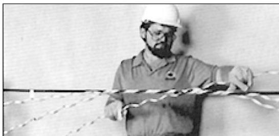
**STEP 6** To complete application, wrap unapplied subsets into previously applied subsets or use both hands to wrap subsets simultaneously into position as shown below. First wrap one end, then wrap the other end. To assure a strong reinforcement, make sure that rods are not crossed and that all rods are evenly spaced. **MAKE SURE ALL ROD ENDS ARE IN PLACE.** Do not use tools that can damage the cable jacket.
