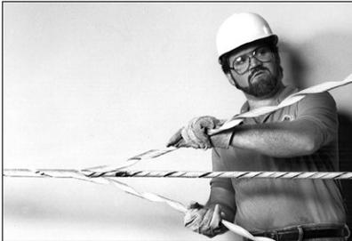
**STEP 9** To ease final installation, do not apply the last two leg pitches. Split the legs as shown below, then apply them completely. Make sure all rod ends are snapped into place.
