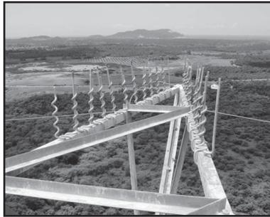
**Step #1** Spread the vertical uprights of the Bird Perch Deterrent and ensure that the helical upright is on the vertical side of the structure angle iron.
