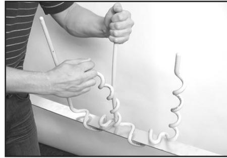
**Step #6** Wrap the helical upright of the second deterrent around the straight upright of the first deterrent. Ensure that the bottom helical wrap is installed properly.
