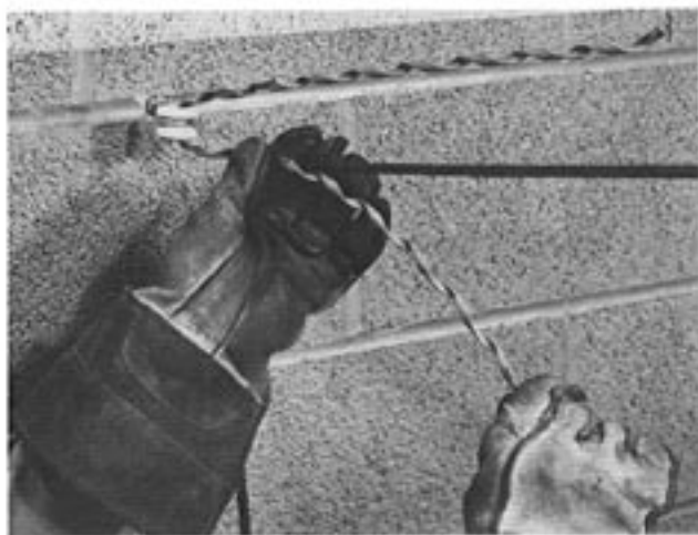
Dead-end as received by lineman in field. Tags indicate proper size and material. Crossover marks aid in application and identification.
