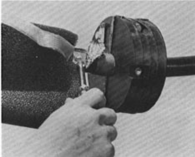
FIGURE 28 - INSERTION OF BONDING BRAID INTO BONDING CLIP - END PLATE INTERIOR
