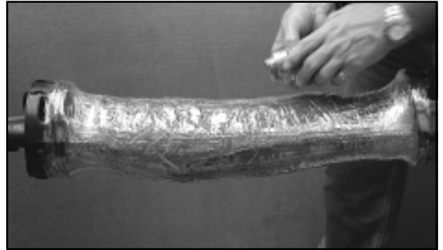
FIGURE 10 - TIGHTLY APPLY 3 OR 4 ADDITIONAL LAYERS OF PRESSURE WRAP TAPE
