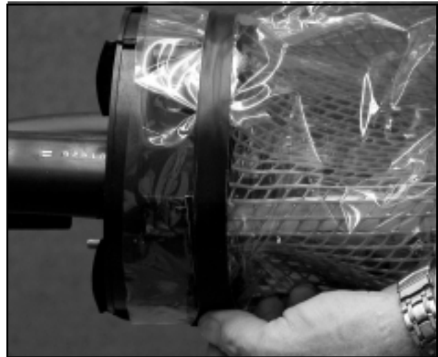
FIGURE 6 - WRAP LOCK-TAPE SEALANT OVER LINER
