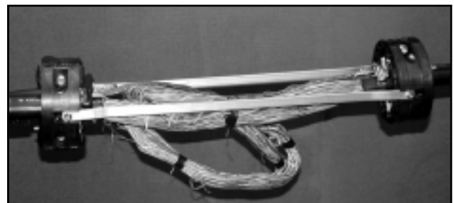
FIGURE 2 - INSTALL TORQUE BARS
