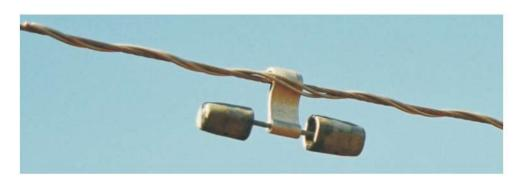
**Application:** The FIBRELIGN® Multi Response Damper is specifically designed for use on ADSS and OPGW and on small diameter aluminium-based power conductors, to control wind induced aeolian vibration, particularly where the fibre optic cable is installed in high voltage environment, typically at 150kV and above.
