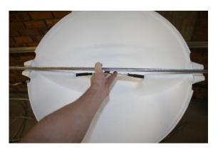
Step 1.5 Keeping the sphere pressed tightly to the conductor, begin wrapping the helical onto the conductor. Ensure the colour mark is to the left/right of the conductor (ie: NOT top/bottom). Repeat for the other side.
