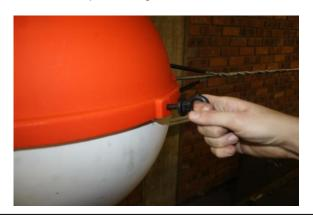
**Step 2.2** Once the pins have been removed, the helical ties can be safely removed and the sphere replaced as per the installation procedure.
