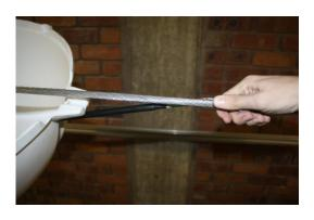
**Step 1.6** Seat the other half of the sphere on top of the installed section ensuring the base and locator tags are aligned correctly. Repeat step 1.5, wrapping the helical ties on to the conductor.
