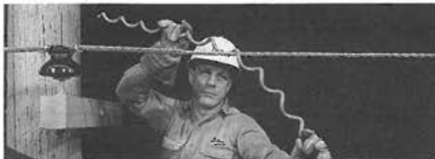
Spiral Vibration Damper or Dielectric Damper as received at job site.
