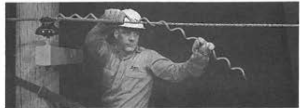
Spiral Vibration Damper or Dielectric Damper as received at job site.
