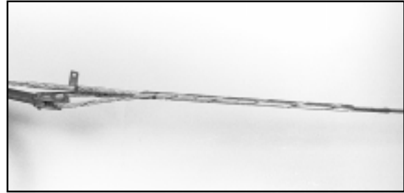
FIGURE 16 - FINISHED APPLICATION OF DEAD-END
