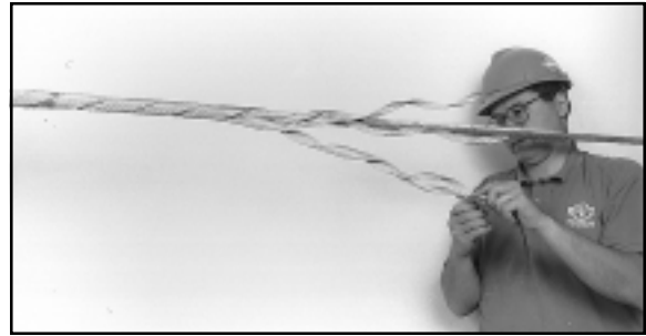
FIGURE 15 - SPLIT LEGS TO EASE APPLICATION
