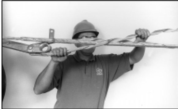
FIGURE 13 - MATCH DEAD-END CROSSOVER MARK AT SRR COLOR CODE MARK
