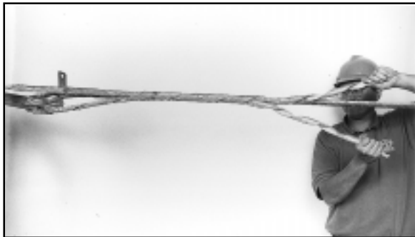
FIGURE 14 - WRAP LEGS OF DEAD-END
