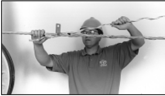
FIGURE 8 - ALIGN SECOND SUBSET WITH CURRENT TRANSFER TAB
