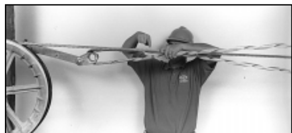
FIGURE 2 - POSITIONING DEAD-END COMPONENT
