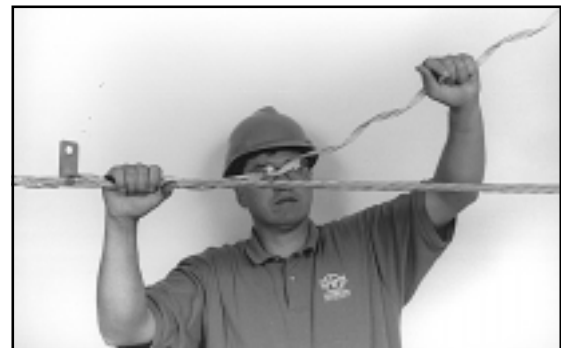
FIGURE 7 - APPLY FIRST SUBSET BY WRAPPING UP AND AWAY FROM CABLE
