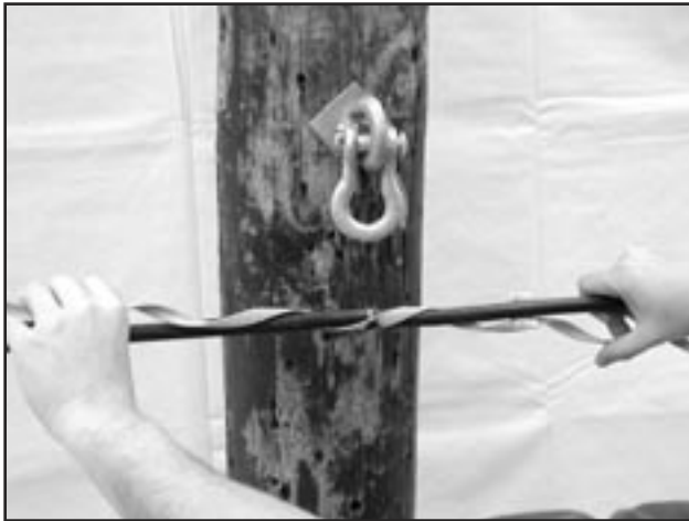
FIGURE 13 - ALIGN FIRST SUBSET
