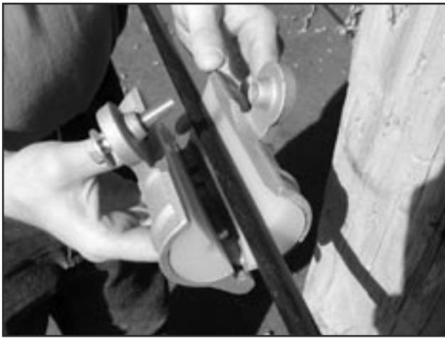
FIGURE 9: LAYING CABLE INTO GROOVE OF INSERT
