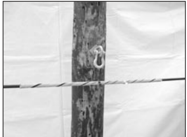
FIGURE 15 - STRUCTURAL REINFORCING RODS INSTALLED
