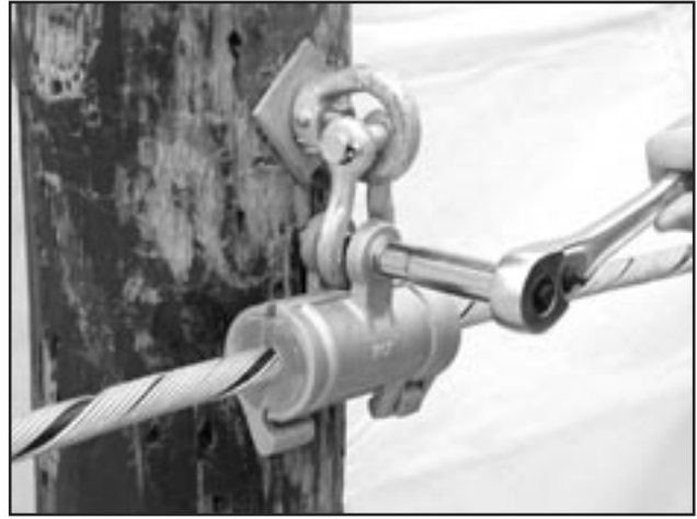
FIGURE 18 - WRENCH TIGHTEN - FLATTEN LOCK WASHER
