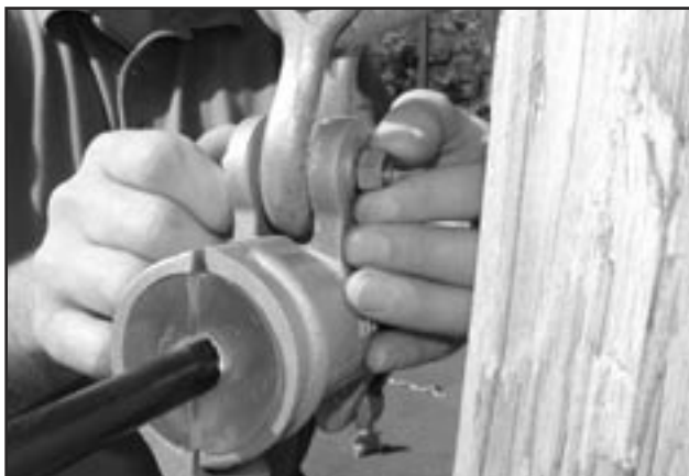
FIGURE 10: INSTALL LOCK NUT
