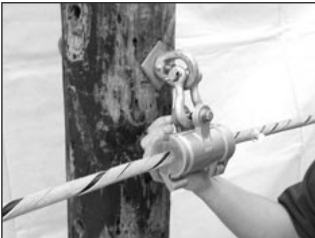
FIGURE 17 - INSTALL LOCK NUT
