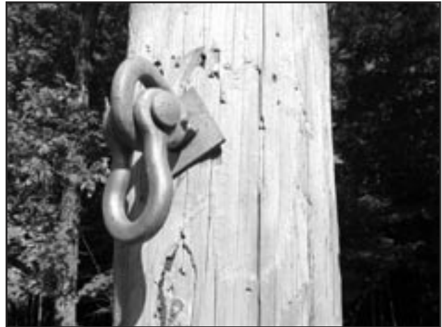
FIGURE 4 - EYE NUT 5/8" & ANCHOR SHACKLE OPTION
