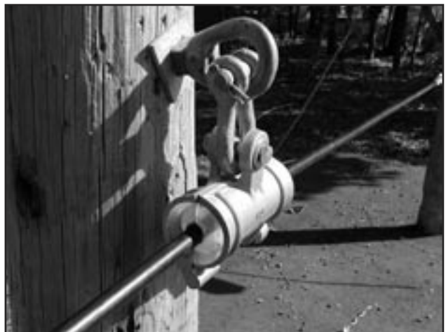
FIGURE 5 - FASN INSTALLED WITH EYE NUT 5/8" & ANCHOR SHACKLE OPTION
