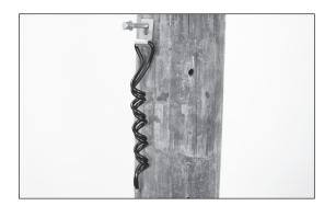
**Step #3** Begin wrapping the first pitch nearest the bracket of the Riser Cable Support around the cable.
