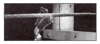
8.00 After Tap Protection Rods are completely installed, wire brush and apply an inhibitor to the surface of the rods in the area where the tapping clamp is to be attached. Repeat this procedure each time the clamp is removed and reattached.
