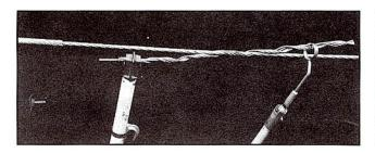
12.00 Prepare the conductor before applying rods. With the rod-ends on the top of the pin as shown in picture #11, begin the application by applying at least one wrap of the subset with an Applicator Ring as shown.
