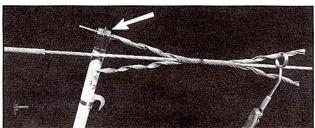
13.00 With the rod ends of the second subset on the bottom of the pin, as shown by arrow, the subsets phase properly. Align the center marks and begin the application of the second subset. After both subsets have been started, work them alternately out to the ends.
