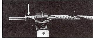
11.00 Insert pin into subset, then clamp with hold stick. NOTE: Rod-ends are positioned on top of the pin.
