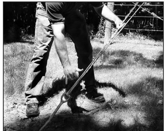
**Step #3** Wrap a leg of the GUY-LOCK on the main down guy installing at least 2-3 pitches.
