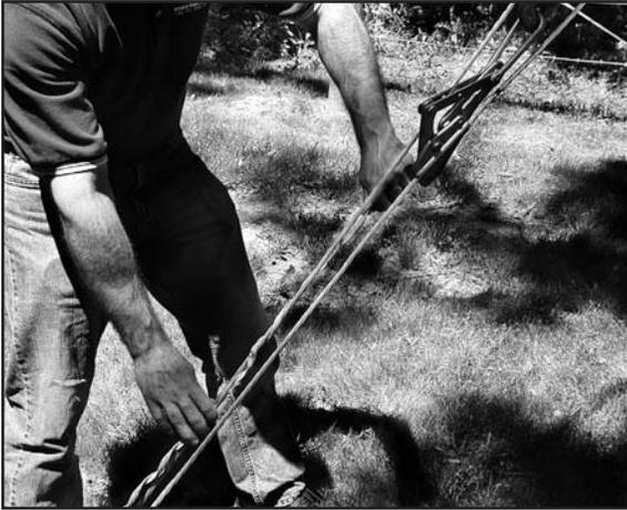
**Step #4** Next, gently squeeze the strand together at the color code location. Wrap the second leg on the tail side of the strand, wrapping toward the hardware.
