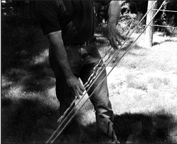
**Step #1** Once the desired tension is achieved, install the first subset on the main down guy and wrap at least 2-3 pitches.
