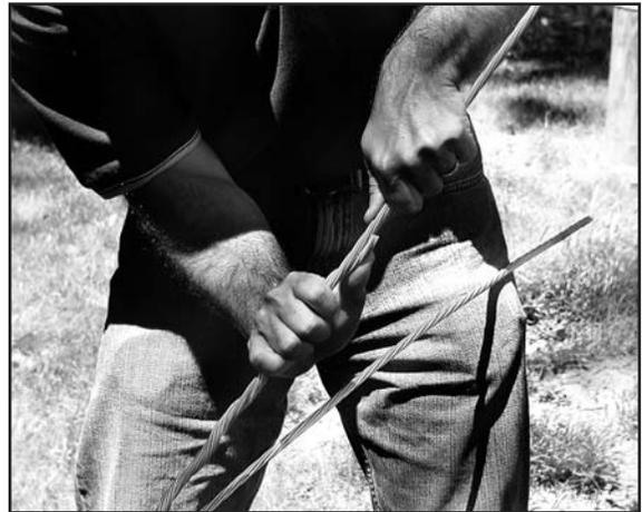
**Step #7** To complete the installation, cut the excess strand at the desired location and secure the tail to the main down guy.
