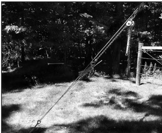
**Step #2** Once the desired tension is achieved the GUY-LOCK is ready to install. First, lay the GUY-LOCK over the main down guy (not the tail portion).
