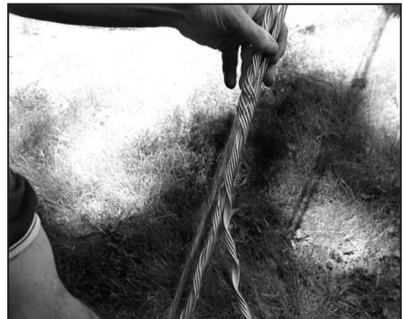
**Step #5** Finish wrapping the second GUY-LOCK subset until the rod ends are completely installed.
