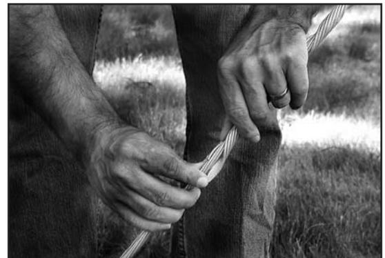
**Step #6** Remove the come-a-long and the Chicago grips from the strand. Finish installing both legs of the GUY-LOCK. Ensure that all rod ends are completely snapped in place.
