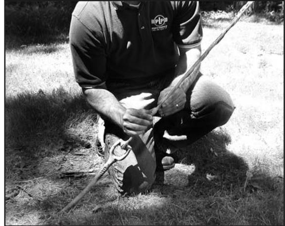
**Step #6** Next, remove the come-a-long and Chicago grips from the strand. Finish installing the first leg of the GUY-LOCK. Ensure that the rod ends are completely snapped in.
