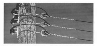
Completed application of PREFORMED Dead-End: Coated
