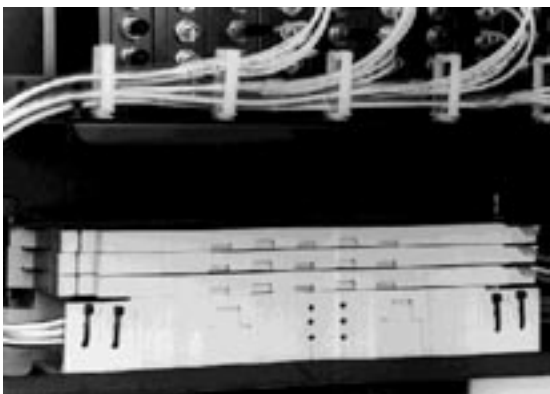
FIGURE 15 - SECURE SPLICE TRAYS WITH SPLICE TRAY HOLD DOWN STRAP
