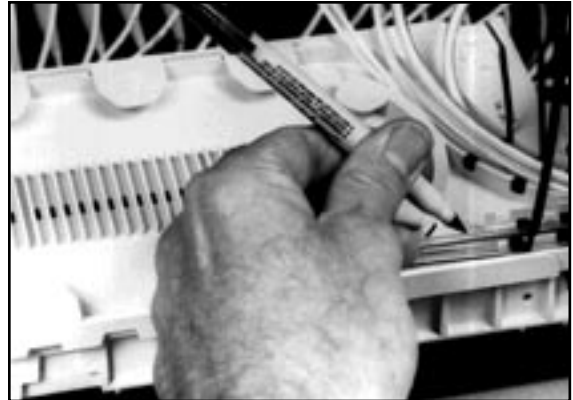
FIGURE 12 - MARKING TUBES IN SPLICE TRAY
