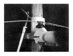
6) With the PREFORMED Applicator Ring start to wrap on one leg of the Distribution Tie
