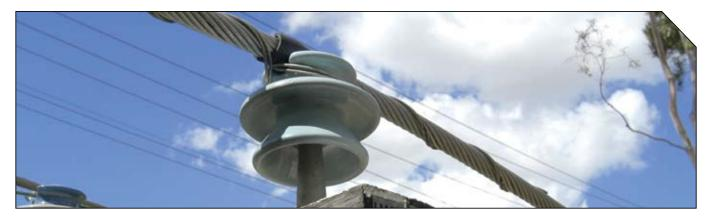
Distribution Ties are designed and manufactured to secure conductors in the top groove of insulators.
