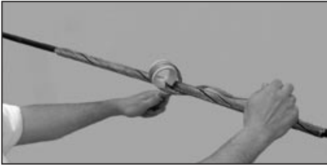
FIGURE 11: WRAPPING OF THE FIRST LEG OF THE MIDSPAN CONNECTOR
