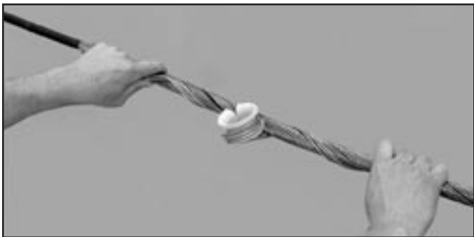
FIGURE 12: WRAPPING OF THE SECOND LEG OF THE MIDSPAN CONNECTOR
