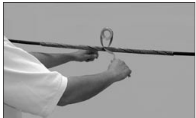
FIGURE 10: ALIGNMENT OF MIDSPAN CONNECTOR
