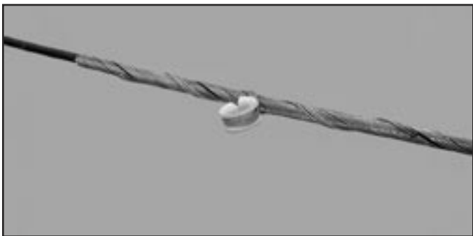
FIGURE 13: COMPLETED INSTALLATION OF THE FAMD
