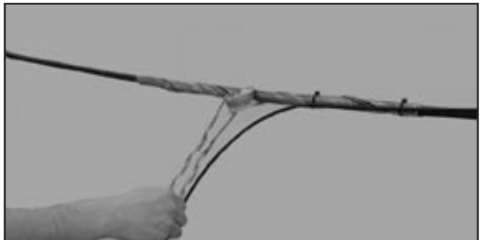
FIGURE 15: INSTALLATION OF DEAD-END ON FAMD
