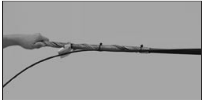
FIGURE 14: INSTALLATION OF TIE WRAPS
