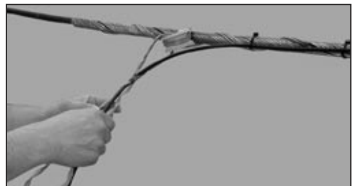
FIGURE 16: BEGIN WRAPPING AT DEAD-END CROSSOVER MARKS
