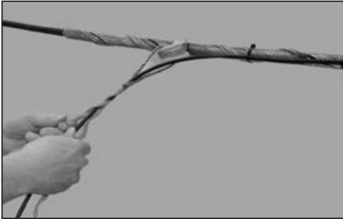
FIGURE 17: WRAPPING LEGS OF DEAD-END
