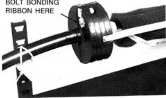
Figure 31 — Insertion of Bonding Ribbon into Bonding Clip—End Plate Exterior
